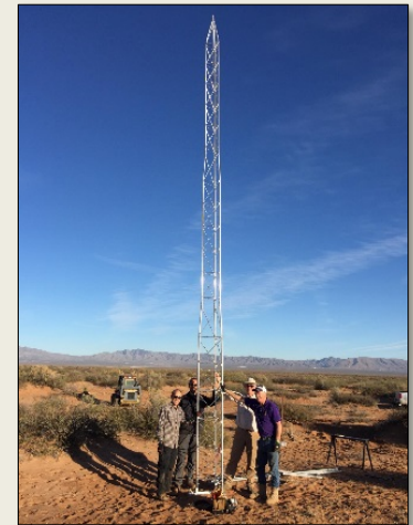
1 st tower installed 1 Dec 2016
